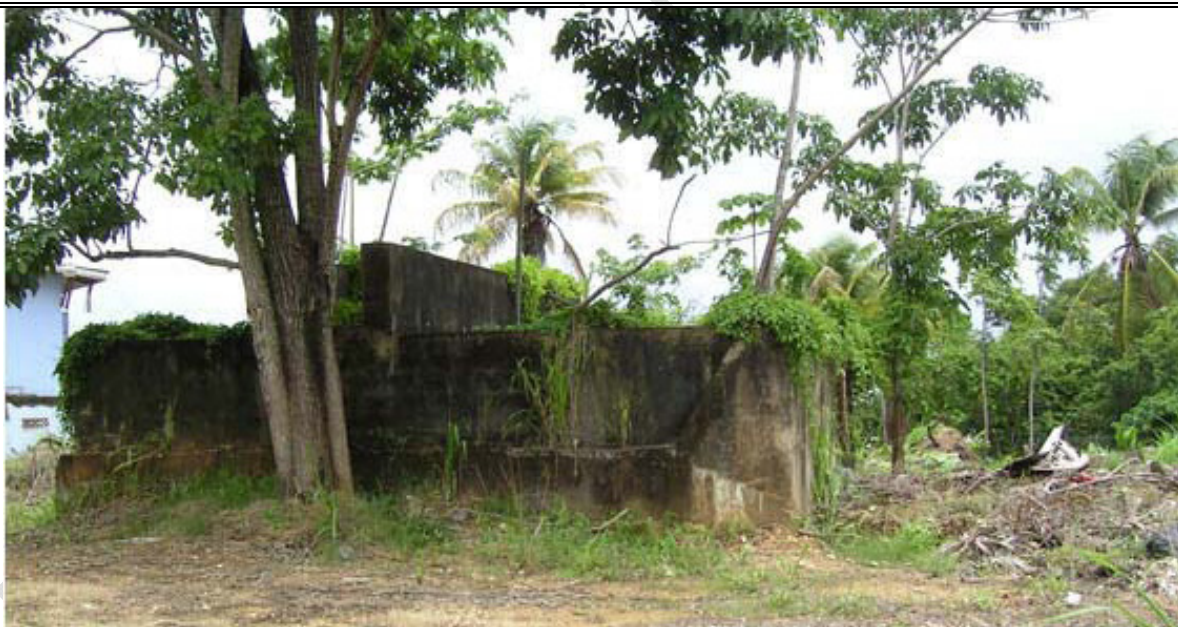
PHOTOGRAPH 2-1: CONCRETE WWTP AT BREGON PARK (2007) (SOURCE: GENIVAR CONDITION ASSESSMENT REPORT)
